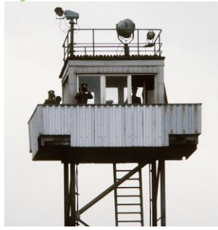
Architecture and material of tower & ladder
